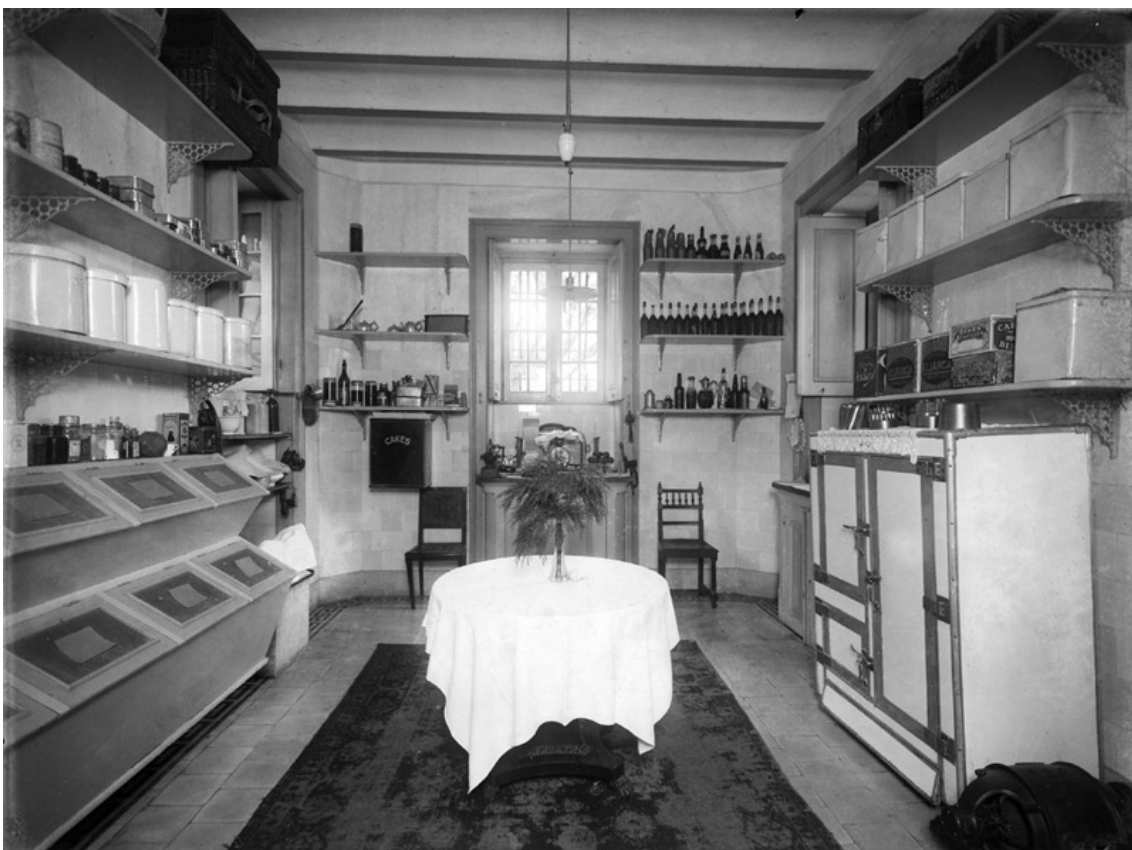
Fig. 4 - Mansion Silva Graça. Kitchen on the basement 20
