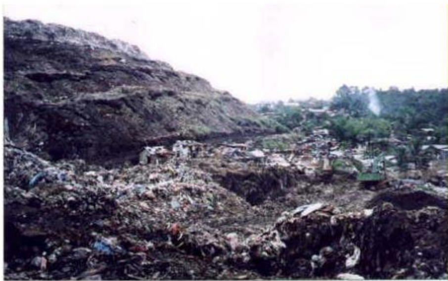
Figure 7: Collapsed slope on the day after the failure
